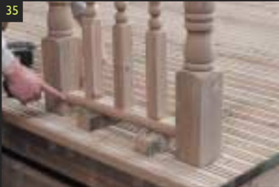
35 Use supports to help ensure the rail is level. Make sure there is sufficient space to fit the bottom angle brackets. Ensure the gap between the deckboard and base rail is no greater than 100mm.
