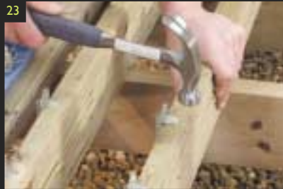
23 Nail the deck clips to the leading edge of the board. Space the deck clips about 50mm from each joist.
