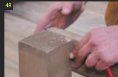
48 Ensuring the back rail is square with the newel post fix using two or more galvanised or stainless steel screws.
