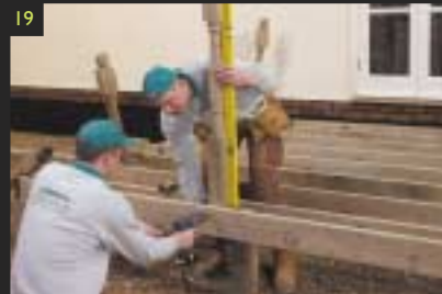
19 Ensure the newel post is vertical and attach it to the inside of the beams with landscape screws or coach bolts. Repeat this process around the inside perimeter of the deck, spacing the posts at a maximum of 1800mm centres.
