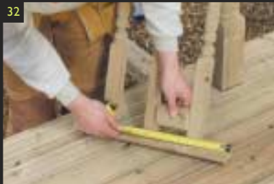
32 Use a spacer to ensure that the spindles are evenly spread. The maximum gap between the spindles must be no more than 100mm.
