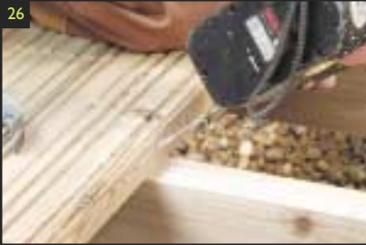
26 Skew screw through the side of the deck board to attach the board to each joist. If necessary pre-drill at the ends of the boards to prevent splitting.
