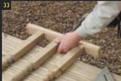
33 Lay the spindles flat and attach the bottom rail using the galvanised or stainless steel screws.
