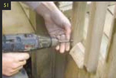
51 Calculate the spacing required on each spindle (max 100mm) and attach using a spacer as a guide.
