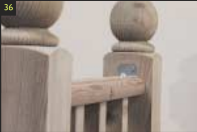
36 To prevent the top bracket being seen, fix the bracket so the vertical plate is above the top rail.
