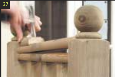
37 Gently knock the finished rail into place. Use an offcut to prevent damage to the rail.
