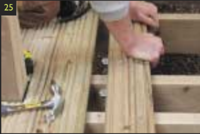
25 Push each board against the previously fixed board. The deck clips should fit under the fixed board. They should give a minimum of 3mm gap between the boards.
