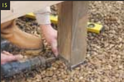
15 Where possible make sure the original treated end of the post is on the ground and attach using galvanized or stainless steel screws.
