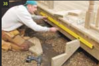
38 ADDING THE STEPS Mark the level along the length of the side beam.
