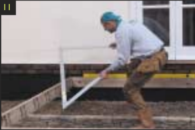
11 Check the beams are square using a 3, 4, 5 square, reinforcing all the corners using a framing anchor.
