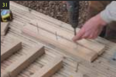
31 Starting from the centre mark the position of the spindles on the handrail. For easier fitting start the screws in position on the rail before attaching the spindles.
