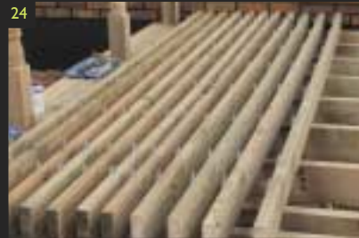
24 For speed of fitting prepare several boards in advance.
