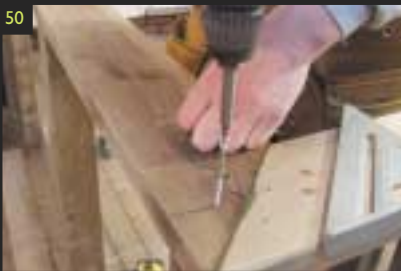
50 Cut the next piece of handrail at 45 degrees, butt to the original piece and fix using screws or deck rail ties.
