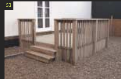
53 The finished deck fitted with the Arbordeck contemporary handrail.
