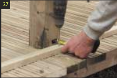
27 Once all the boards are fixed, determine the position of the edge of the deck. Attach a baton as a temporary guide line.
