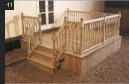
44 The finished deck fitted with the Arbordeck classic handrail. The sides of our deck have been cloaked with deck boards. Adequate ventilation has been provided to allow the substructure to dry after rain.
