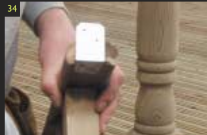
34 Fix the brackets using the screws provided.
