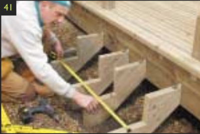
41 Attach additional stringers to ensure the maximum distance between them is no more than 400mm on centre.
