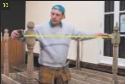
30 ATTACHING THE SPINDLES AND HANDRAIL Using a tape, measure the distance between the newels on the handrail and cut to length.
