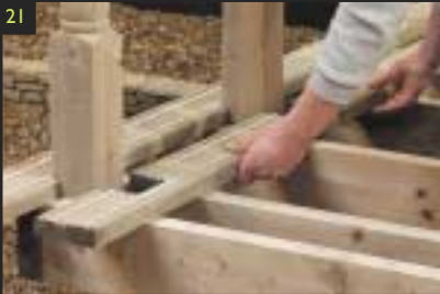
21 When notching the boards leave a 2 - 3mm gap around the post to allow for movement of the boards.
