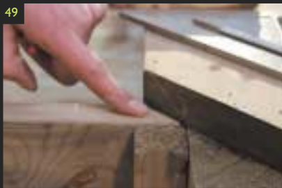
49 Cut the end of the top rail at a 45 degree mitre (for a 90 degree join) and fix using screws or deck rail ties.
