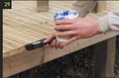
29 Don't forget to brush the cut ends with End-grain.
