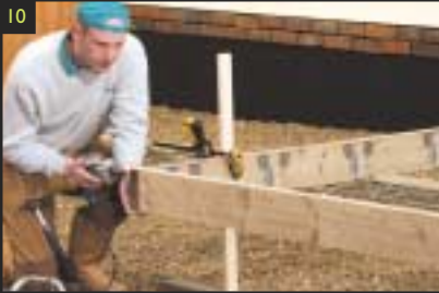
10 Attach the end beam using landscape screws.
