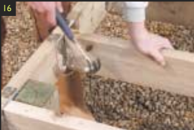
16 After treating the cut ends of the joist with End-grain, nail in place into the joist hanger. If you are using the contemporary handrail system you can now start to fix your deckboards.
