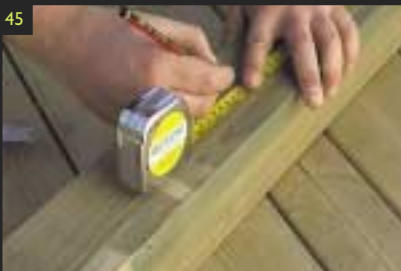
45 The top of the handrail should be 900mm from deck level. Mark this height on the newel post.
