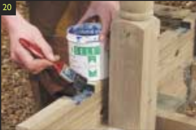
20 LAYING THE DECK BOARDS After carefully marking the boards notch out positions for the posts and treat with End-grain.
