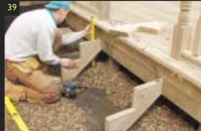
39 Checking for the vertical attach the furthest stair stringers.
