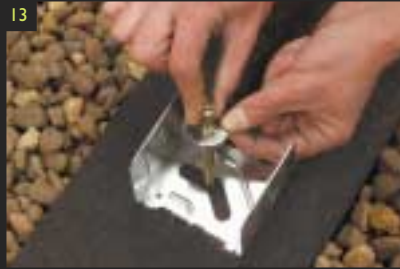
13 Accurately position the post bases and attach using expanding bolts.
