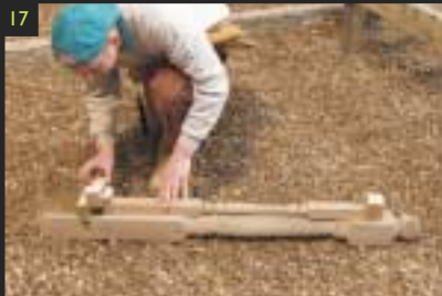
17 ATTACHING THE NEWEL POSTS Calculate the height of the handrail by placing all the components on the newel post. Mark the height of the top of the joist.
