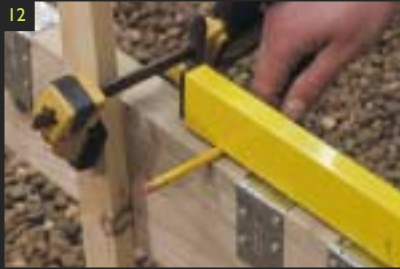
12 Adjust the height of the side beams to allow a slight fall in the deck away from the house. This will ensure the deck drains correctly.
