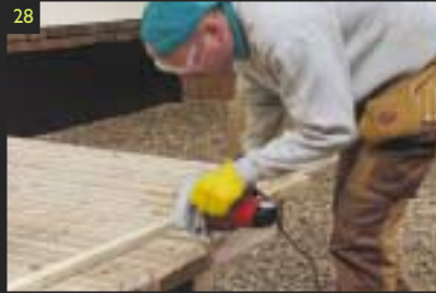
28 Using the guide line trim the excess board with a circular saw. Remove the guide baton.
