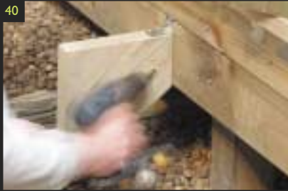
40 Secure the stringer by skew screwing to the beam or using a framing anchor.
