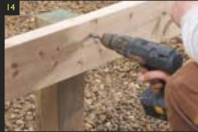
14 Attach the posts to the beams using coach bolts or landscape screws.
