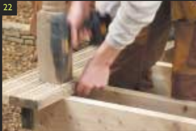
22 Attach the first two boards by screwing through the surface using galvanized or stainless steel deck screws.
