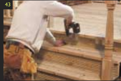
43 Starting from the bottom fix the boards by screwing through the face into the stair stringers.
