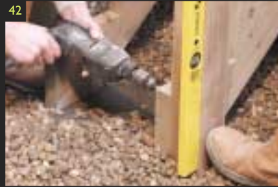
42 Holding the newel post vertical attach using landscape screws. Remember this post is resting on the ground and so should be supported by a concrete pad and post base.
